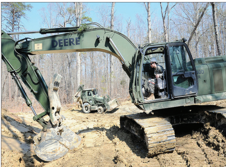
Sgt. Nathan Goff with the 207th Engineer Company works on a drainage ditch at Camp McKee, a Boy Scouts camp in Montgomery County, Ky., April 9, 2014.
