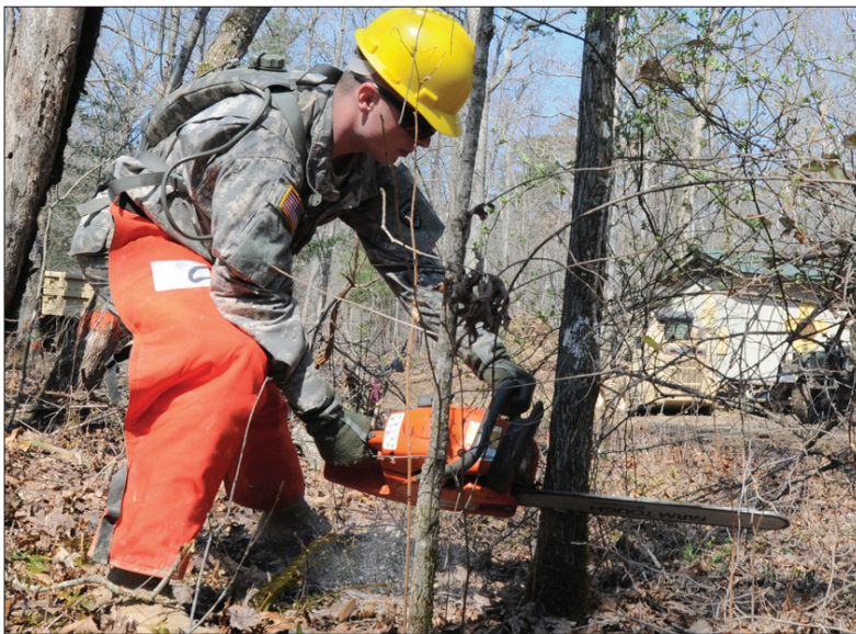
Pfc. Matthew Joseph with the 207th Engineer Company uses a chainsaw to remove trees to expand a parking area at Camp McKee, a Boy Scout camp in Montgomery County, Ky., April 9, 2014.
